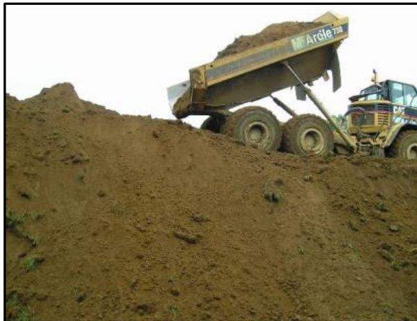
Figure 20. Stockpiling of topsoil.
